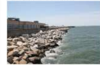
Sea Wall and Riprap
