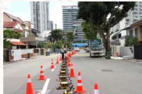
Between Road Lanes
