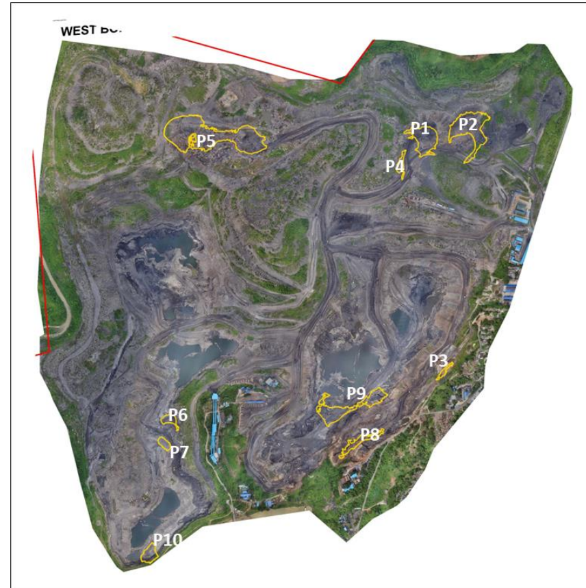
Drone data analysis from 1 st – 30 th September. Polygons represent dumping area during the period
