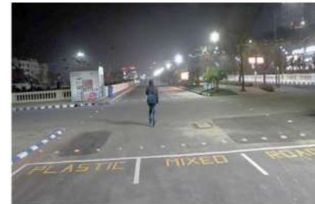
Plastic Road (using 850kg of plastic waste)
