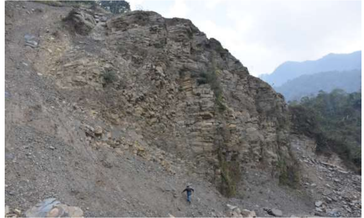
Photograph showing close joints in the thinly bedded sandstone. Little disturbance makes the rock crumble down because of the closely spaced joint and bedding planes
